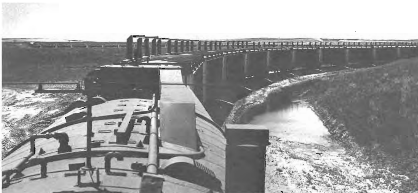
Consist of unit coal train snakes around loop spur at Gascoyne, N. D. mine as it moves in for loading.
