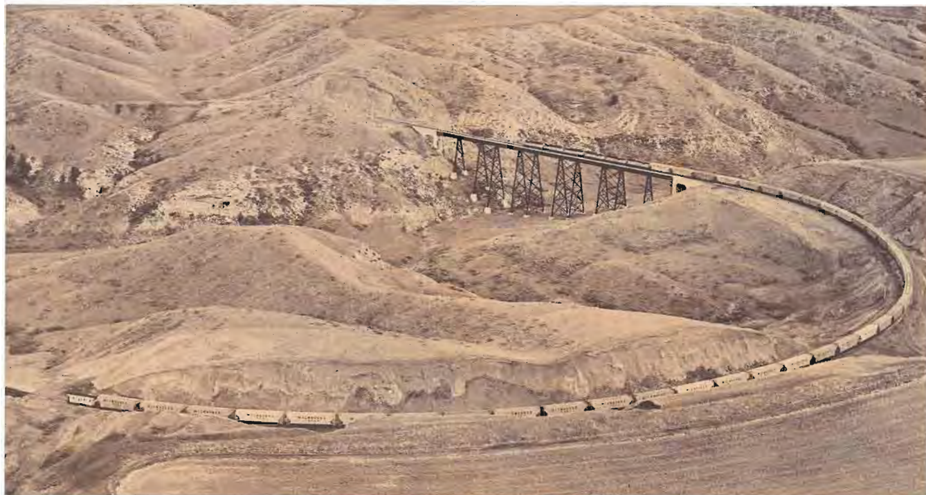
A trainload of wheat moving in Milwaukee Road covered hopper cars crosses Red Coulee Creek trestle near Waltham, Mont.
