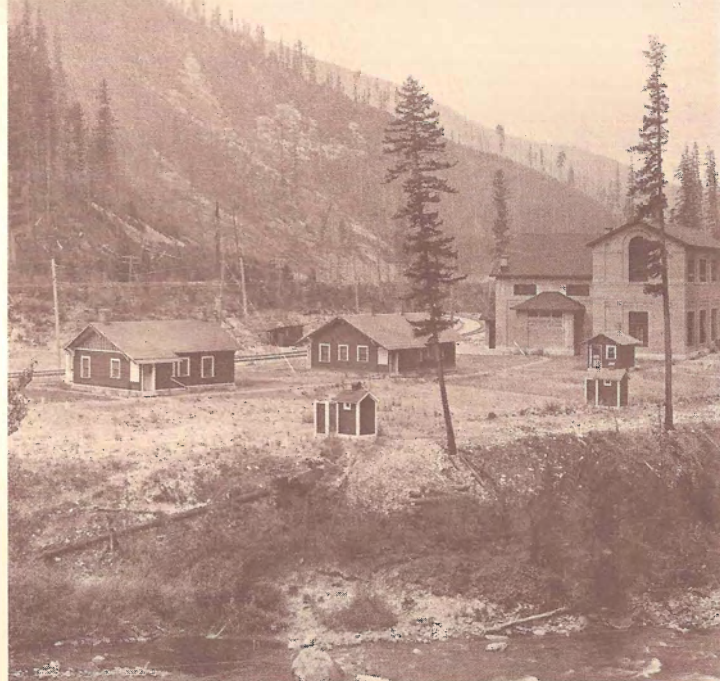
The substation and residences at Drexel, Mont. are shown as they looked shortly after their construction in 1916. Twenty-two such installations were built along the electrified portion of track to convert the 100,000 volt A.C. delivered by the power companies to the 3,000 volt D.C. required for electrified operations.
