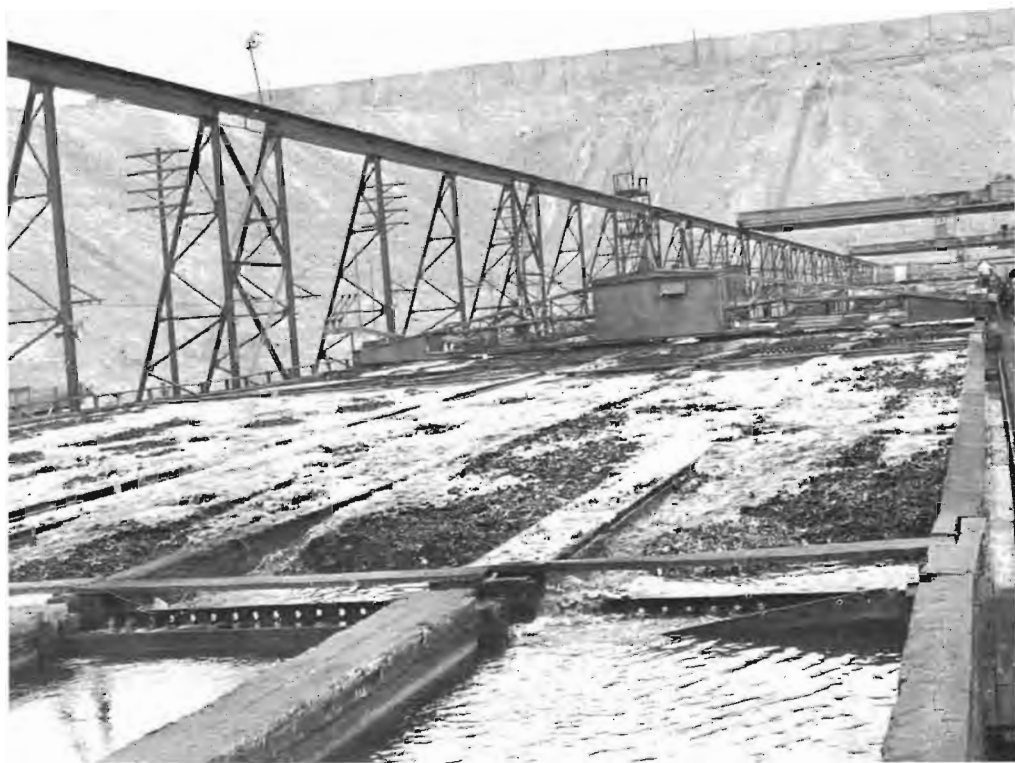
The precipitation plant contains eight launders (long canals in which copper is precipitated) separated into six sections each. The scrap is spread evenly in each launder section and the copper solution is piped in. The resulting chemical reaction forms copper that is nearly 80 per cent pure.
