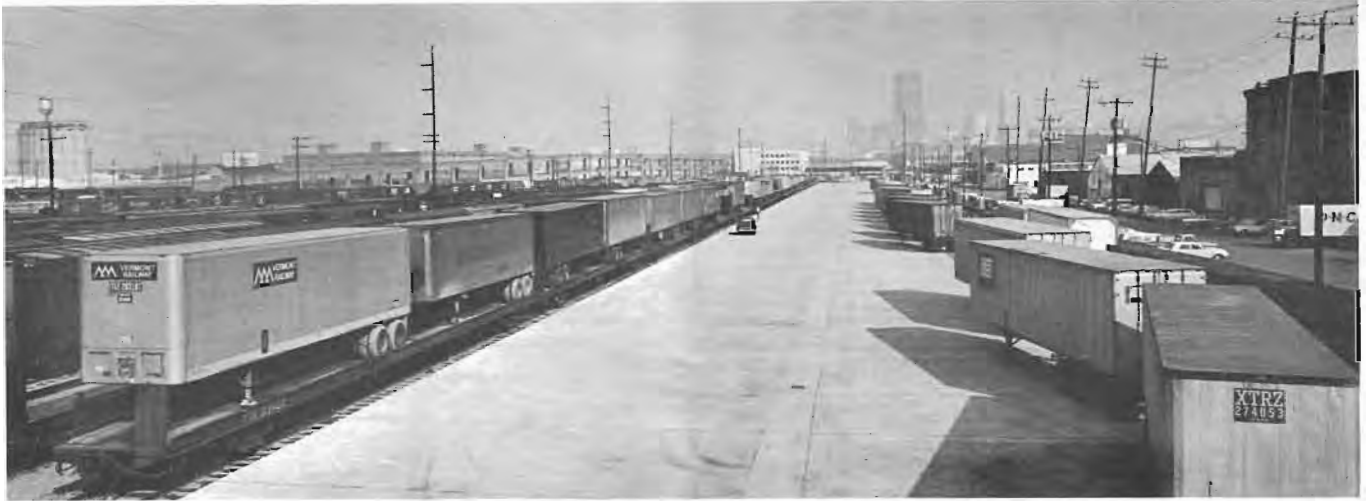
A three-block long concrete apron is the backbone of the newly modernized and expanded piggyback/container yard.
