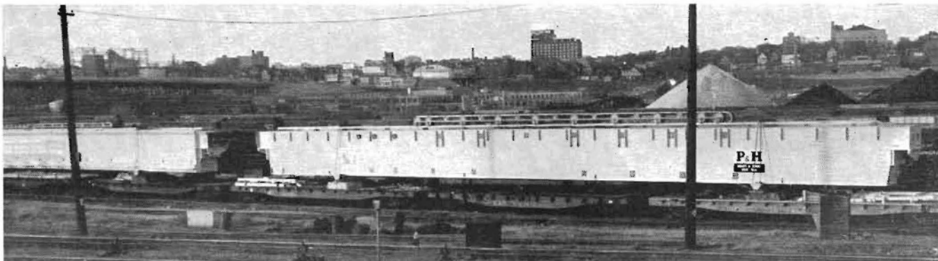
The first of the huge overhead cranes for the new multi-million dollar Jones & Laughlin steel mill at Hennepin, Ill., ready
