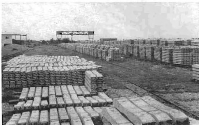
Stores of concrete ties manufactured in the railway's own plant, which also turns out pre-stressed concrete bridge girders.
