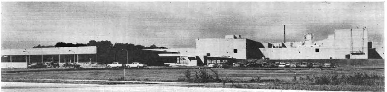
The new 250,000 square foot plant, the largest chocolate and cocoa producing facility in the Midwest, viewed from a
