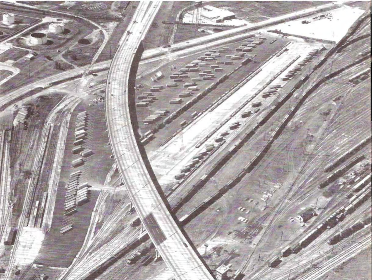
Aerial view in a southwesterly direction showing the full expanse of Piggyback Park, the Milwaukee Road's greatly expanded TOFC facility at Bensenville, Ill., and its principal piggyback terminal for the Chicago area. The 46-acre park, newly-paved, newly-lighted and greatly expanded both in area and in trackage, went into full-scale operation on Sept. 19 (see "Roaring '90s" campaign starting on page 4). The facilities occupy the entire area from lower left to the upper right corner, the white triangular part at upper right being the holding lot for hotshot movements. Trackage at lower right is part of Bensenville Yard.
