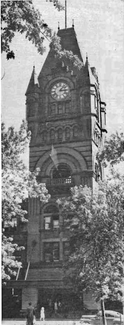
A view of the tower before it was lowered in 1953. The canopy dated from modernization work in 1943.
