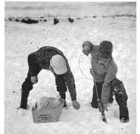
Blasting experts charge cuts with dynamite. Detonation points were located by fence-to-fence measurement.
