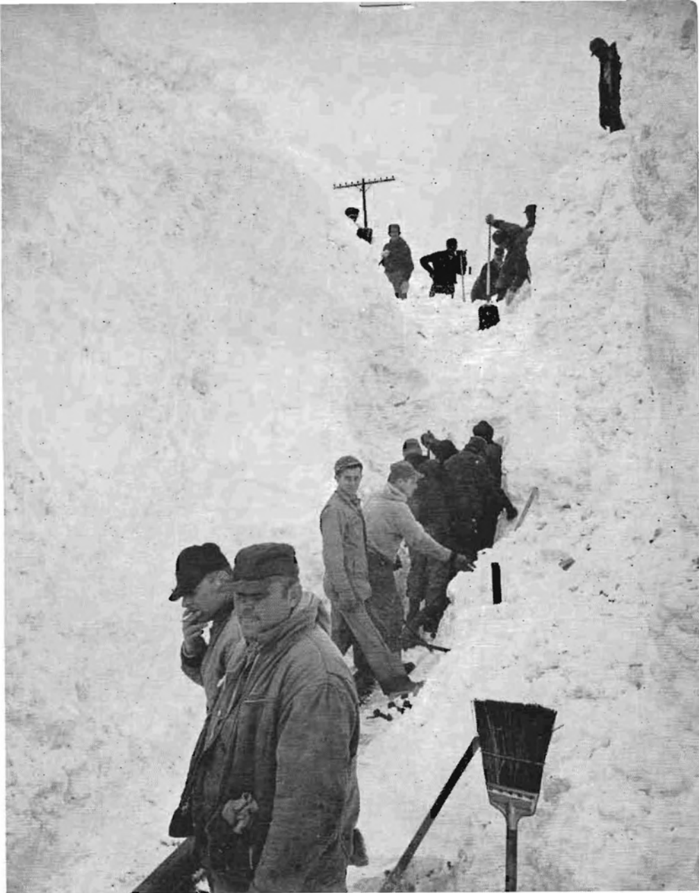
Changing out rail broken by steam rotary in drift at Alamo, S. D., calls for a lot of shoveling.
