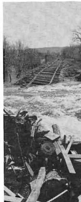
RECORD SNOWS fed the ravaging spring flood waters that inundated and washed out sections of our railroad in the Mississippi Valley from St. Paul, Minnesota to Muscatine, Iowa.
