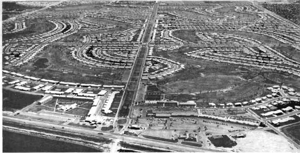
Aerial view of Sun City's motor hotel and shopping center (foreground, left and right), and some of the homes and apartment units adjacent to the two 18-hole golf courses.
