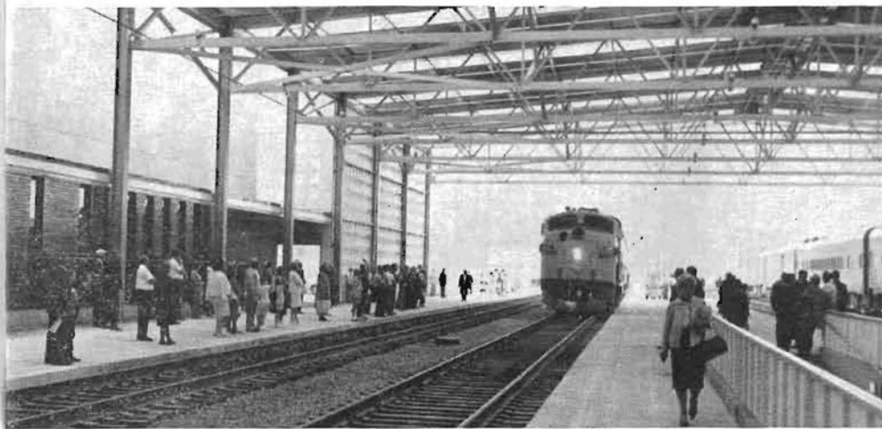
Scene as the first train into the new terminal arrived on the morning of Aug. 4. At right is one of four ramps connecting with the tunnel through which passengers have access to the station.
