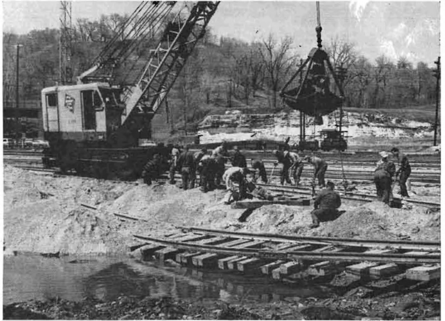
Crews raising and rebuilding track west of the St. Paul roundhouse as the flood tapers off. Final dressing of tracks in the classification yard will continue for some time.
