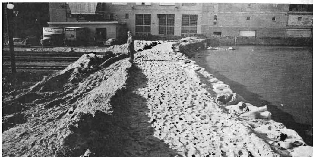
Dike approximately 8 feet high which was constructed over our main and yard tracks at St. Paul to the river retaining wall.
