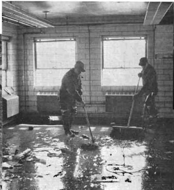
Having hosed the floor of the St. Paul yard office, B&B Foreman E. O. McBride (right) and Carpenter Rayno Hokona remove the remaining muck.
