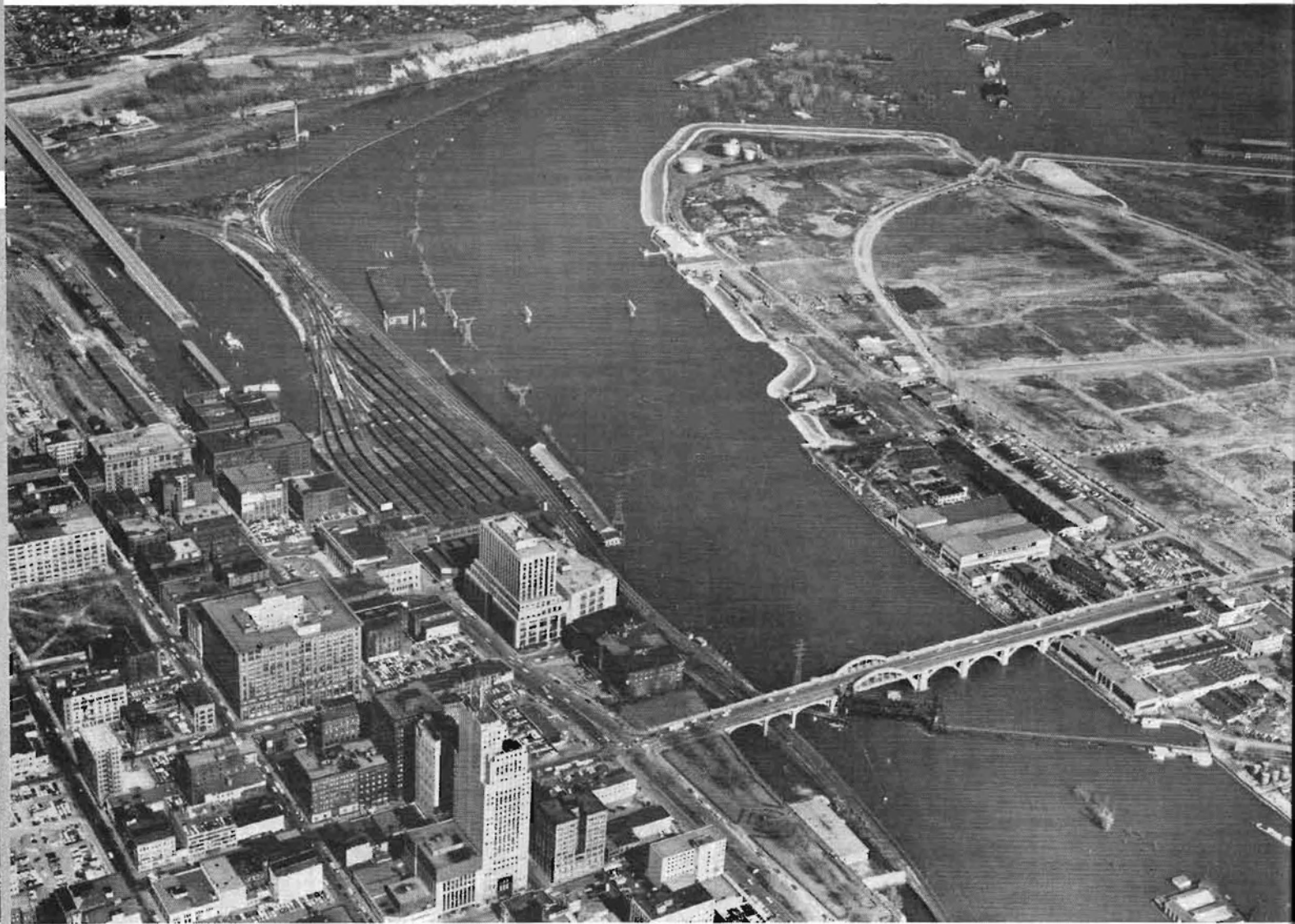
Mississippi floodwaters at St. Paul on Apr. 21 looking east over our main line on the left bank and showing above the Roberts Street bridge the tracks of the Union Station. Isolated buildings at the right of the station tracks are the Sibley Street freight house (front) and the fruit house. Flooded area above the fruit house is our trailer-on-flat car facility under four feet of water.
