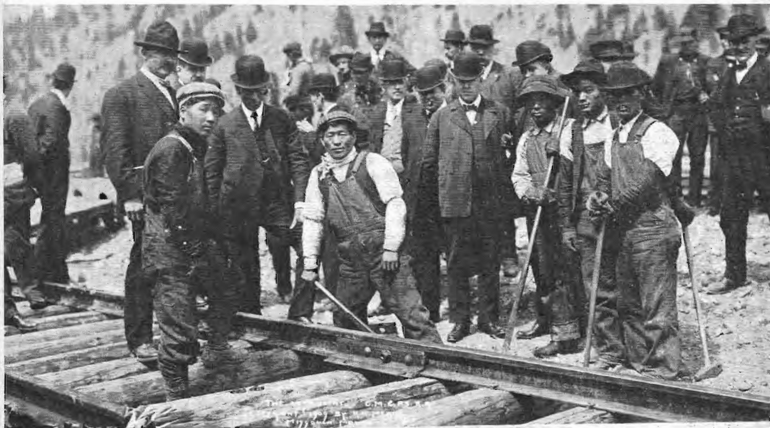
East meets West—installing the last rail joint connecting the transcontinental system near Gold Creek, Mont., on May 19, 1909.
