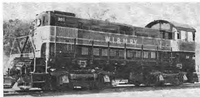
Present day diesel operated on the Washington, Idaho & Montana Railway.
