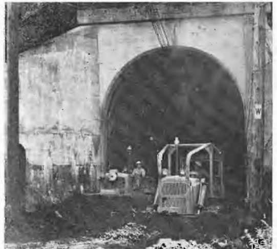
Following blasting and ripping operations in a tunnel, bulldozers remove excavated material. Each pushed toward the machine ahead so the material, in effect, was relayed to the outside.
