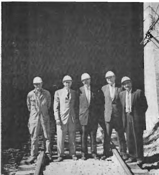
In-the-field supervisors accompanying Chicago headquarters officials on an inspection tour. Posed at the entrance to Tunnel 22 just west of Roland, Ida., are, from left: Rocky Mountain Assistant Division Engineer F. W. Striebel; P. L. Cowling, assistant to president; M. T. Sevedge, superintendent of the Rocky Mountain Division; L. V. Anderson, general manager - system; and R. D. Claborn, division engineer for the Rocky Mountain Division.
