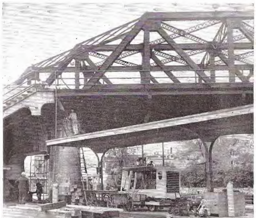
LIFTING A 464-TON BRIDGE. Scene at La Crosse, Wis., showing the Rose Street viaduct which spans the Milwaukee Road's main line and yard tracks west of the depot as it was recently in the process of being raised 6 inches. The engineering feat, a part of the Road's over-all program to provide higher clearances for modern loadings, entailed jacking up the span and inserting steel plates between it and the piers underneath. Here, D. H. Fisher, supervisor of bridge maintenance (left), is standing by as Steel Bridge Erector Robert McCall welds plates on expansion bearings. (La Crosse Tribune photo)
