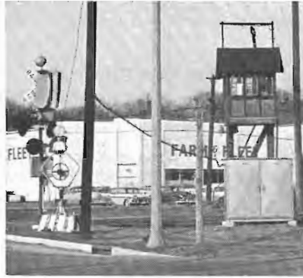
North Humboldt Ave. and East Locust St. in Milwaukee is the crew of R. C. Larsen (top of pole), John Gilbert (right) and Babe Lilla. Above is one of three new signals installed recently at the Five Points crossing in Janesville, Wis., in a joint program with the Chicago and North Western. The old signal tower it replaces was a familiar point on the Janesville skyline for about 100 years. (Milwaukee Journal and Stephen A. Rothman photos)
