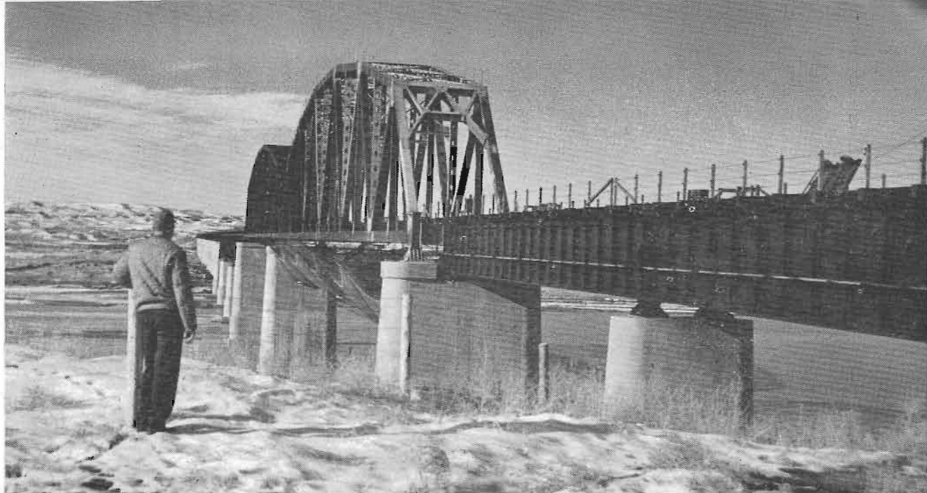
The new Missouri River bridge as it looked shortly before completion. The concrete and steel structure is almost 4,890 feet long.
