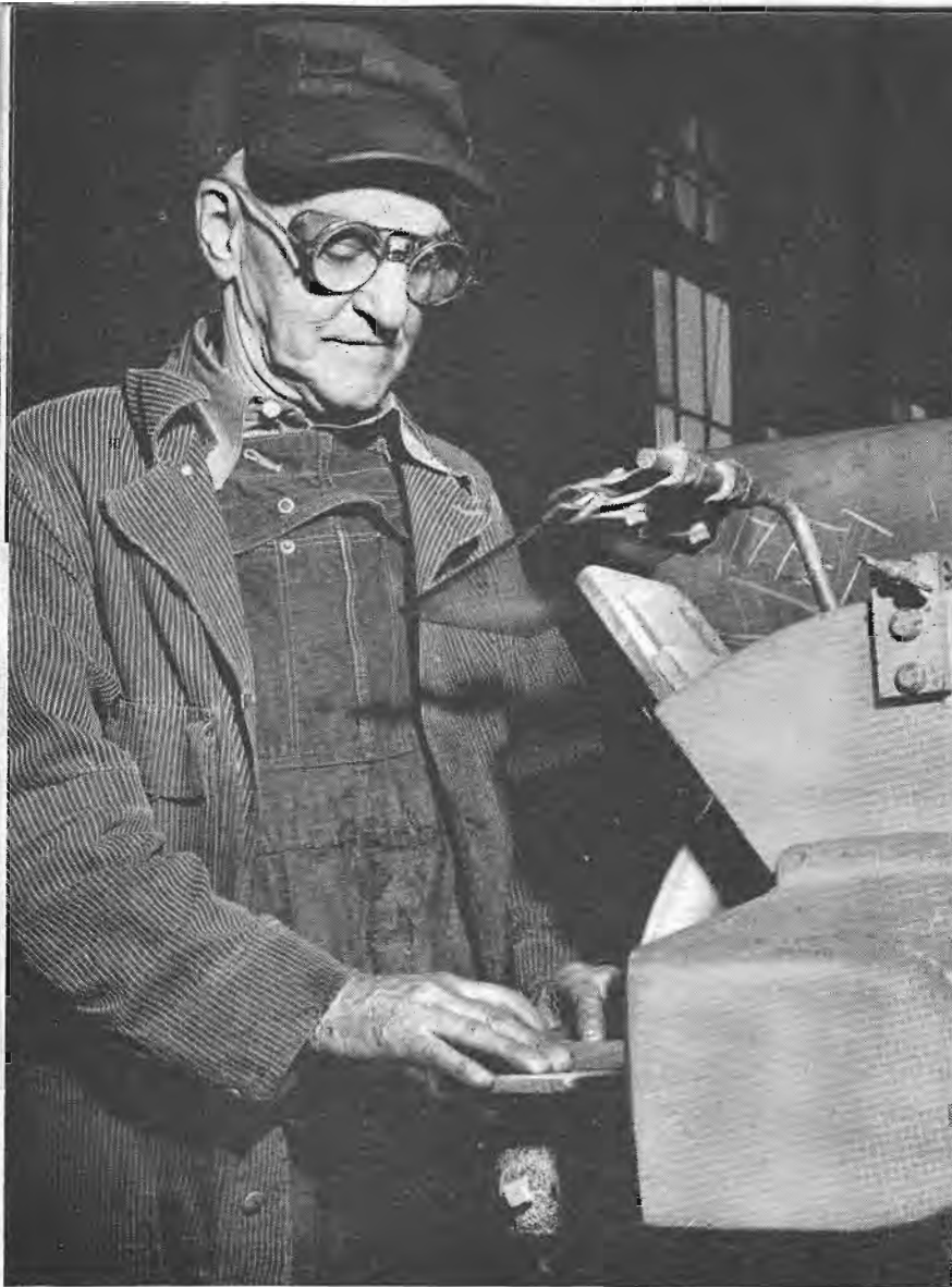
Frank Cauley, machinist in the locomotive machine shop, Milwaukee, wears his goggles at the emery wheel and takes the extra precaution of using the glass shield.
