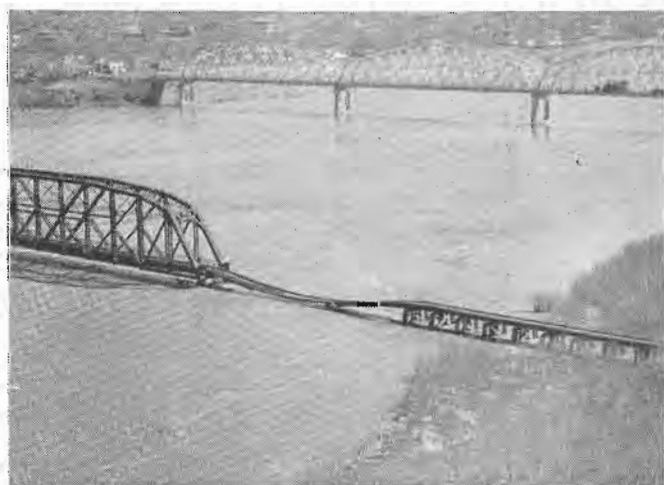
The Milwaukee Road bridge across the Missouri River at Chamberlain, S.D., as it appeared on Apr. 7. The sagging section was later knocked out completely by the pounding of ice carried on the crest of the flood, but was back in service within a few days. (Photo courtesy the Daily Republic, Mitchell, S.D.)
