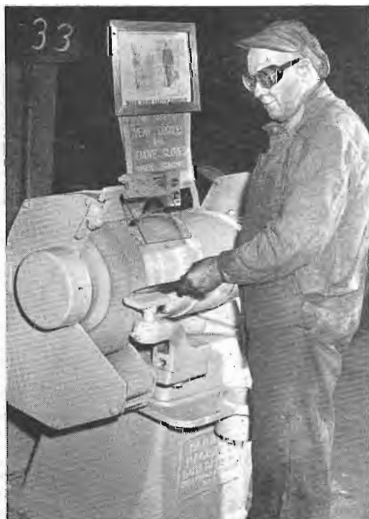
At the Minneapolis roundhouse, one of the firm believers in the importance of wearing goggles is Machinist William Anderson. Note the safety poster above the machine and the glass shield to deflect flying particles of metal. Machinist Anderson takes an active role in promoting the use of safety goggles, serving as roundhouse safety committeeman and also as chairman of the Federated Shop Crafts in Minneapolis.
