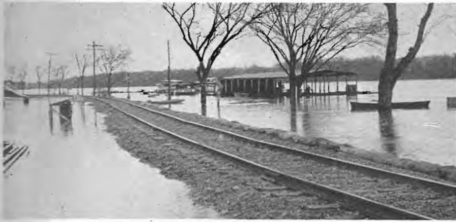
View of the main line through McGregor, Ia., west of the station. The track was raised and sandbagged to keep the trains running. Highway 13, just to the left of the track, is out of sight beneath the flood.
