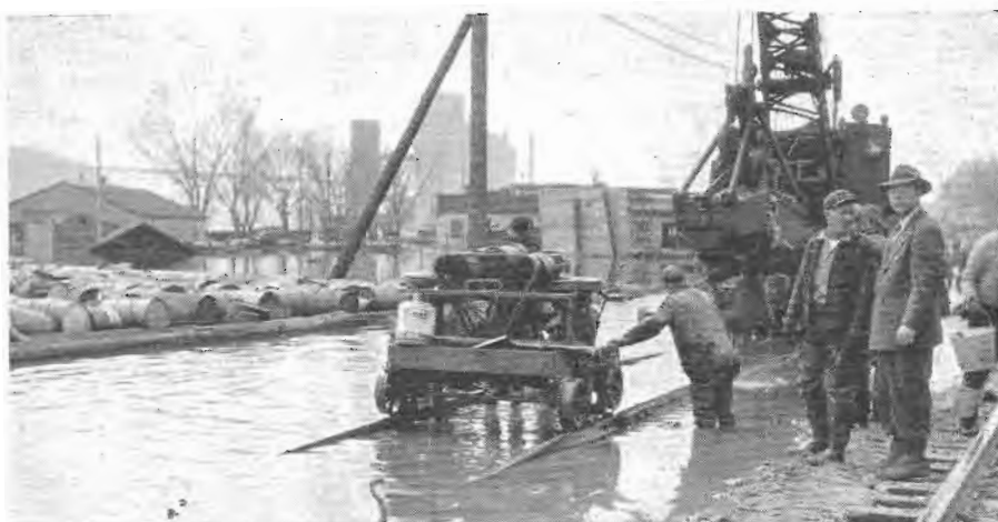
Amphibious operation on the Chestnut Street line, St. Paul, as the eastbound main line was raised. The machine in the foreground is a power jack, used for raising track, while clamshell in the background drops sandbags with which the men filled in beneath the ties. Gravel was later added. At the right, left to right, are J. M. Tracy, general foreman, Section 2, Minneapolis, and L. C. Blanchard, Twin City Terminal roadmaster.
