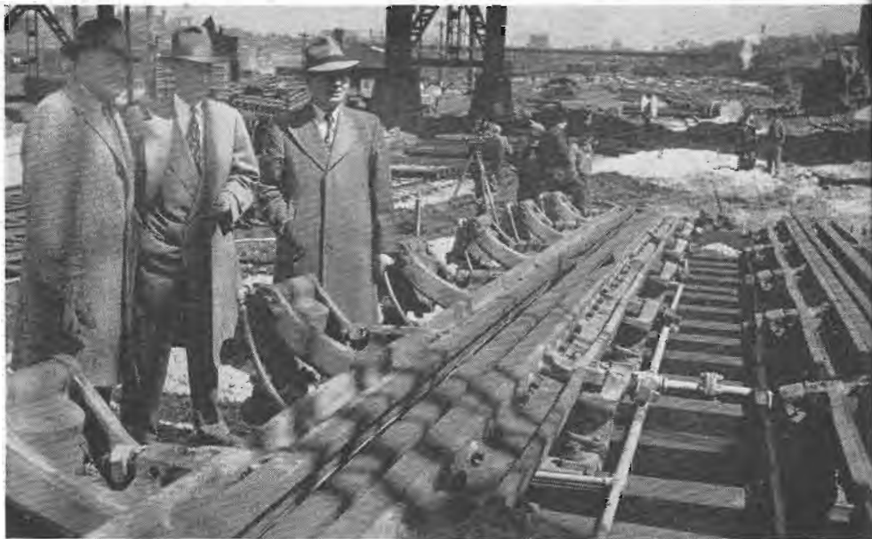
K. L. Clark principal assistant engineer, in charge of field work on the Air Line yard project, J. H. Stewart, general superintendent, Milwaukee, and J. J. Dombrowski, superintendent of the Milwaukee Terminal Division (left to right) study the massive retarder.
