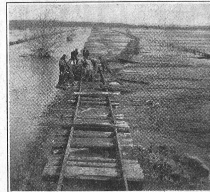
Track Shifted Over the Right-of-Way Fence
