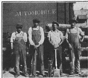
Section Foreman and Crew, Fond du Lac Yard
