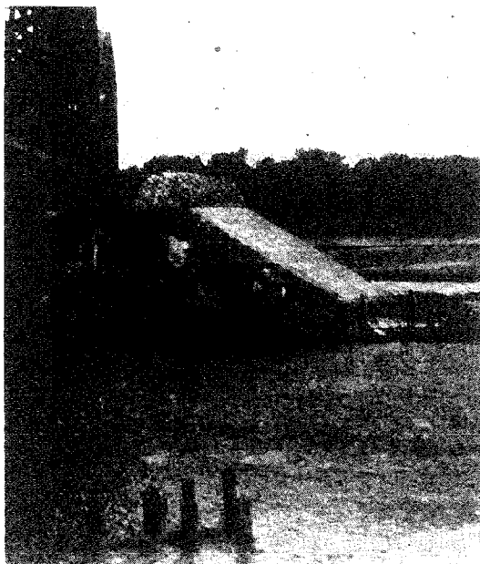
Mat at Pier 3 Looking West
