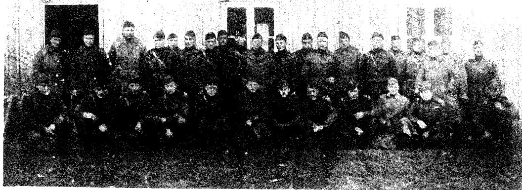
Officers of 13th Engineers Ry. at Fleury-Sur-Aire
