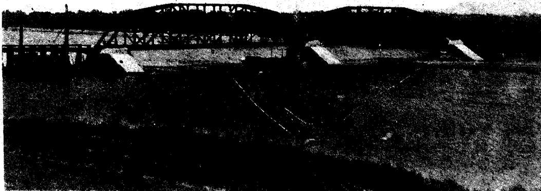
View of Bridge from East Bank.
