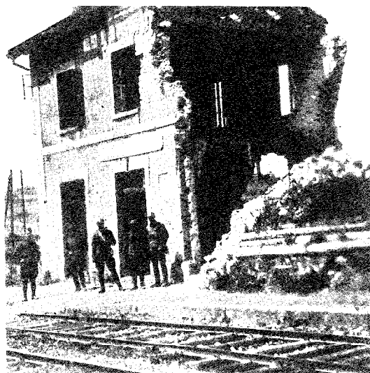
The Ruined Railroad Station of Dombasle, in the Argonne, France.
