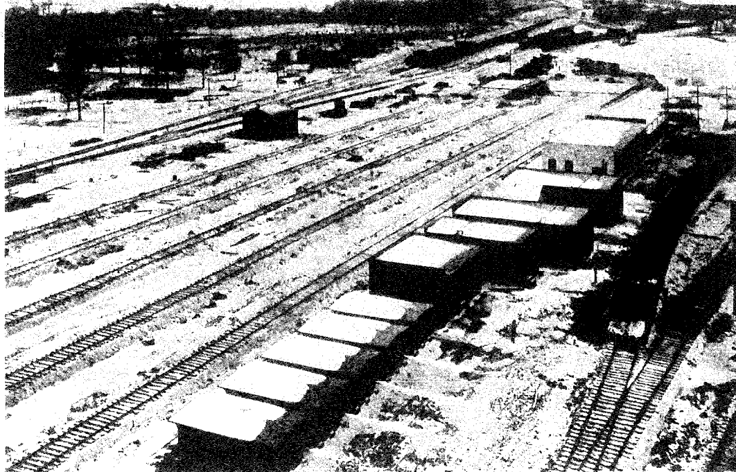
The New Terminals and -
