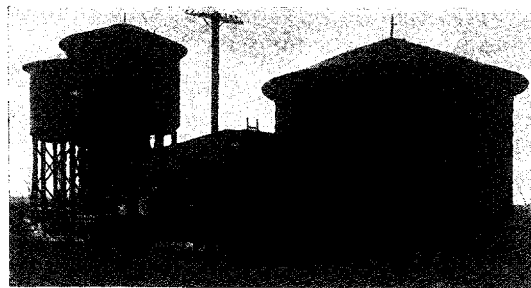
Water Softener and Storage Tanks
