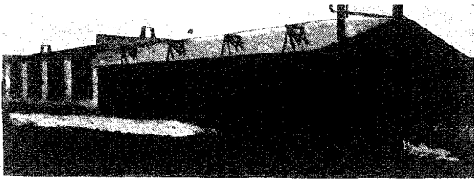
Planing Mill and Lumber Shed, Car Department
