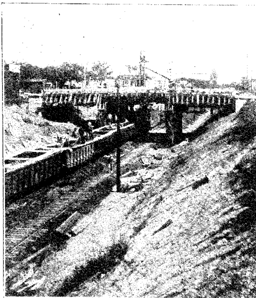
Forms for Concrete Viaducts.
