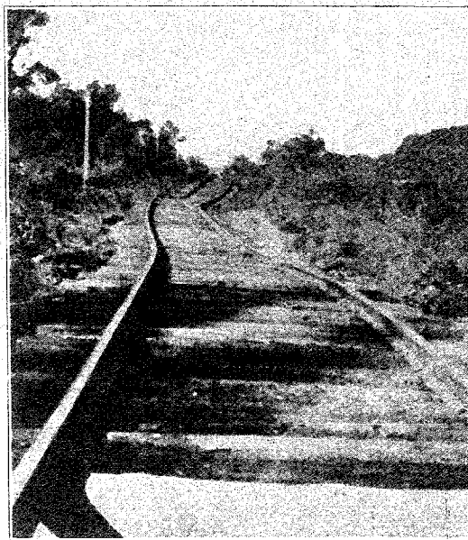
Washed Track, Mineral Point Division.
