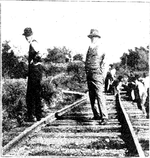
Rebuilding the Track.
