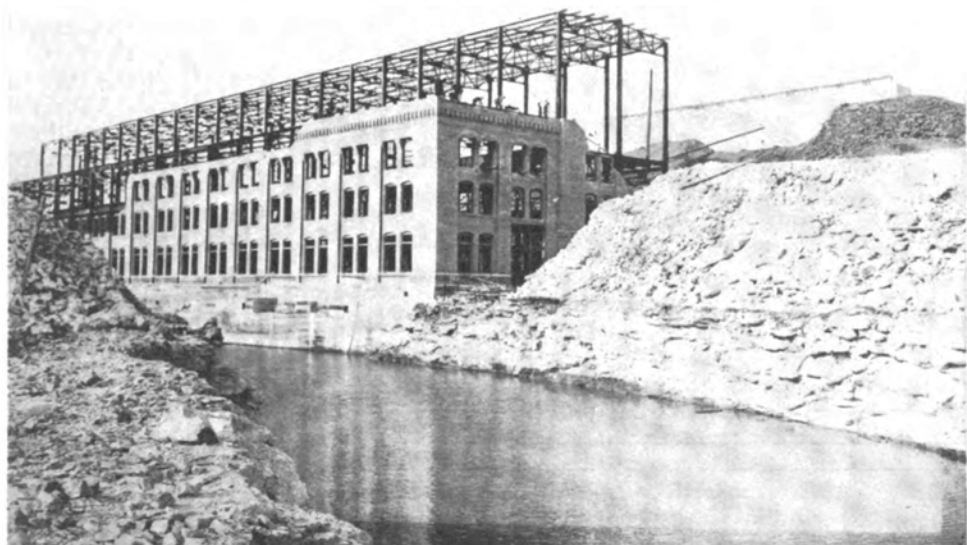
THE POWER-HOUSE, RAINBOW FALLS DEVELOPMENT, IN COURSE OF CONSTRUCTION. IT IS 326 FEET LONG.
