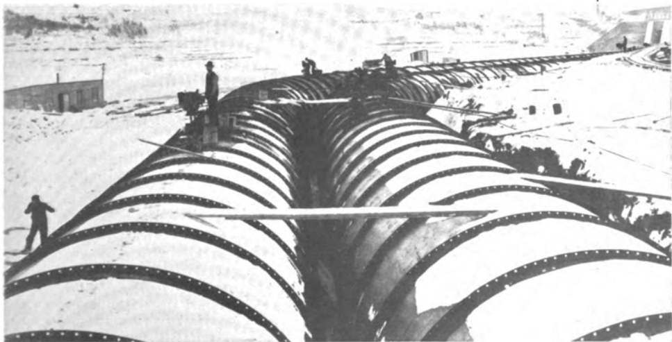
TWO STEEL PENSTOCKS, EACH 15 FEET 6 INCHES IN DIAMETER ONE-HALF MILE LONG, RAINBOW FALLS DEVELOPMENT OF THE GREAT FALLS POWER COMPANY.
