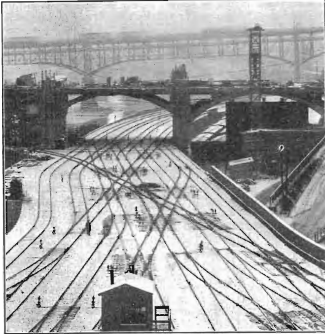
The West Approach
