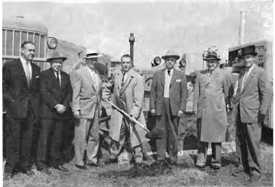
Dignitaries present at the ground-breaking. From left: Frank Gorsh, chairman of the board of county commissioners of Silver Bow County; D. J. Mooney, president of the Cahill-Mooney Construction Co. and vice president of the Butte Chamber of Commerce; T. J. Sullivan, mayor of Butte who was master of ceremonies; C. A. Bradburn, zone manager for Safeway Stores Inc. at Butte; V. E. Straus, assistant general freight and passenger agent of the Milwaukee at Butte; C. H. Steele, western vice president of the Anaconda company; K. R. Coughlin, Milwaukee Road district passenger agent, Butte.
