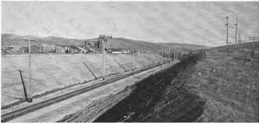
View in an easterly direction at Loweth, Mont., near the west end of the line change, showing the new track. The old line passed the town on the other side.
