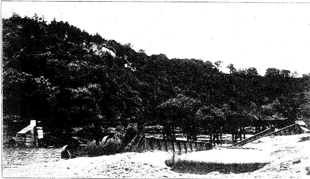
Steel Girder Bridge Wrecked by the Flood.
