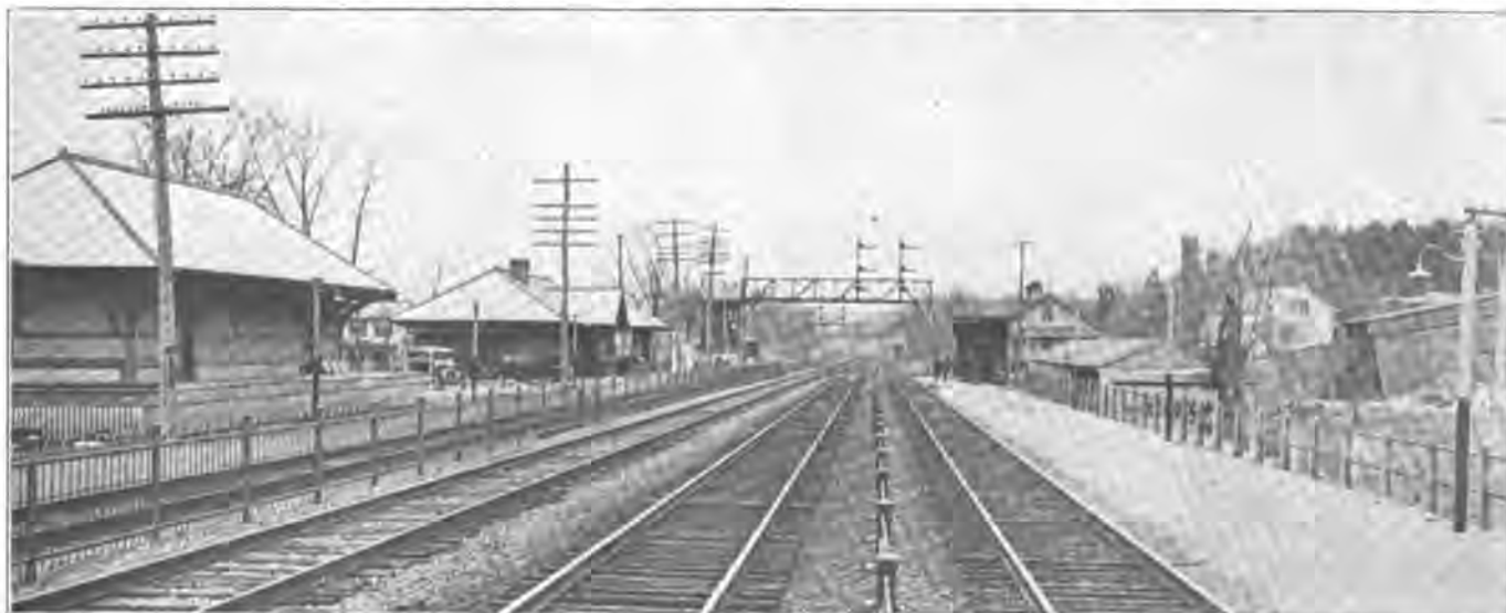
Fig. 1—New Station at Staatsburgh, N. Y., Built in Connection with Four-Tracking Improvements of the Hudson Division, New York Central R. R.
