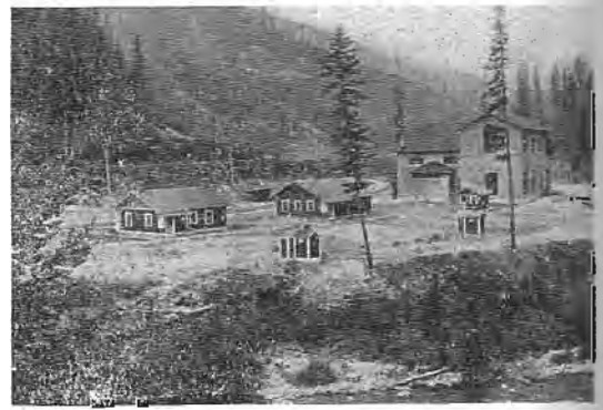
Fig. 2. Substation and Bungalows at Avery, the Western End of the Present Electrification
