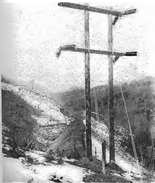
Fig. 3. 100,000-Volt Transmission Tower for Long Span
