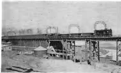
ELECTRIC LOCOMOTIVE DELIVERING ORE TRAIN TO CONCENTRATOR BINS
