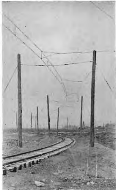
OVERHEAD CONSTRUCTION ON SINGLE TRACK CURVE
