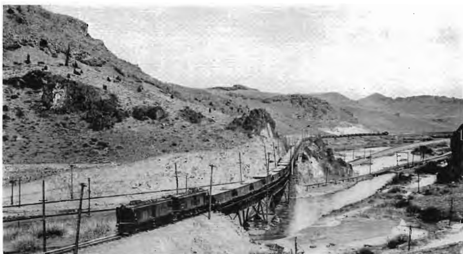
160-TON ELECTRIC LOCOMOTIVE HAULING 4550-TON ORE TRAIN IN SILVER BOW CANYON
