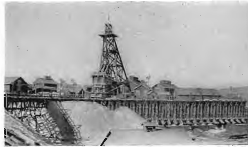
HOIST AND STORAGE BINS ON BUTTE HILL
