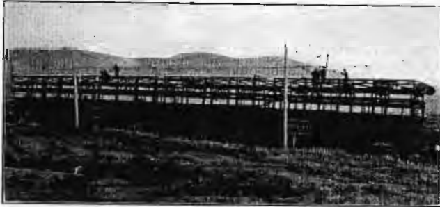
Erecting the Overhead Work
