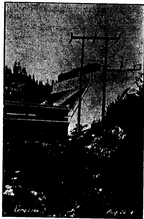
FIG. 5—GATE HOUSE, PENSTOCK AND TRANSMISSION LINE AT LONG LAKE PLANT
