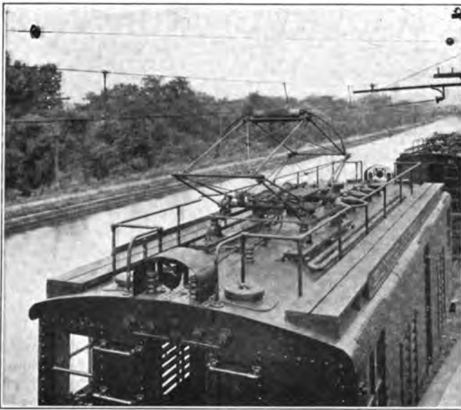
Butte Electrification—View of Apparatus on Roof of Locomotive Cab
