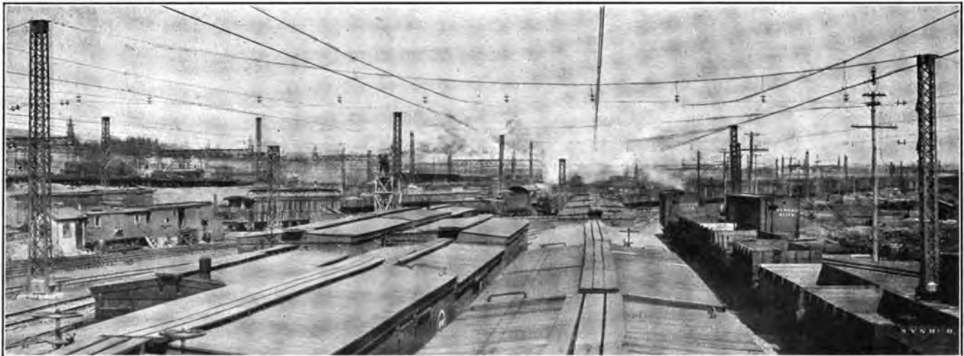
Fig. 5—A.-C.-D.C. Comparison—View of Westchester Yard, New York, New Haven & Hartford Railroad, Showing Simple Overhead Single-Phase Construction
