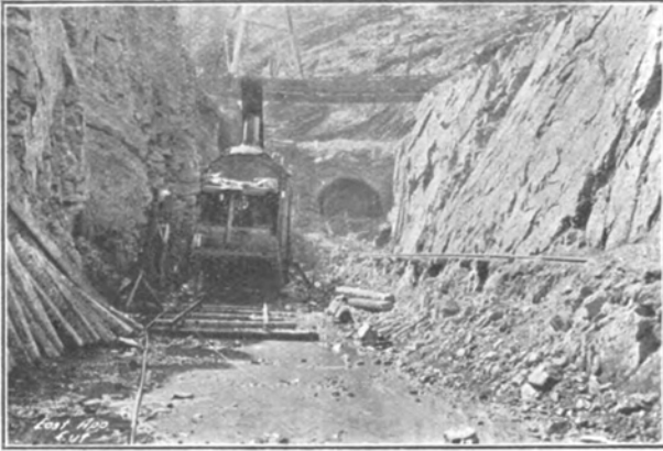
Shovel taking out approach cut at East Portal of St. Paul Pass Tunnel. The East Portal of this tunnel is in Montana, West Portal in Idaho. Heading, at this portal, was started and the muck disposed of by means of a cableway, until the approach cut was completed. Shovel was then put in tunnel and run by compressed air to handle bench-muck.
